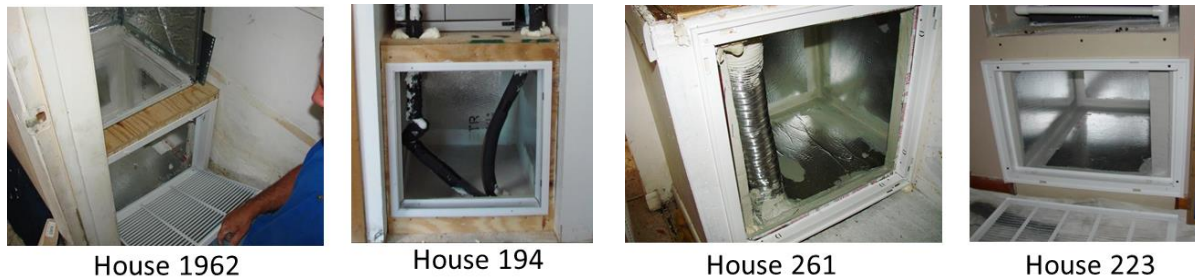
Figure 5-plenums Completed Phase 1 return plenums.
