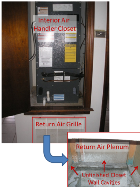
Figure 3. This air handler in an interior closet (left, top) is served by a return air plenum directly beneath (left, bottom) formed by the open, unfinished framing of the closet walls.
